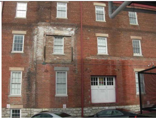
Photo 23- Partial East elevation showing bridge and old canopy
