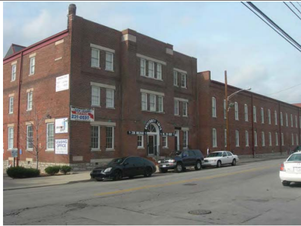
Photo 1 – North Elevation along Bolivar Street is generally in good condition.
