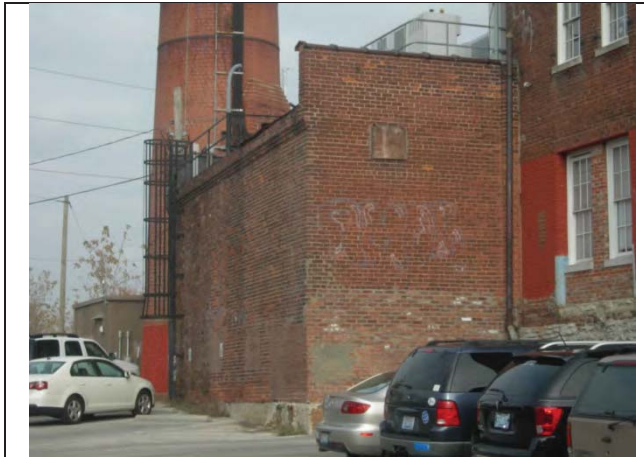
Photo 13- South elevation at old boiler for building.
