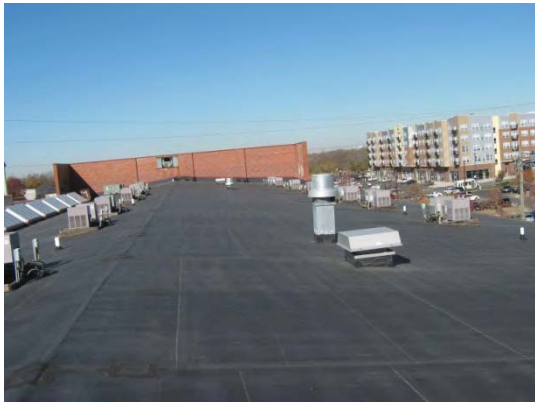
Photo 33- north side of roof
