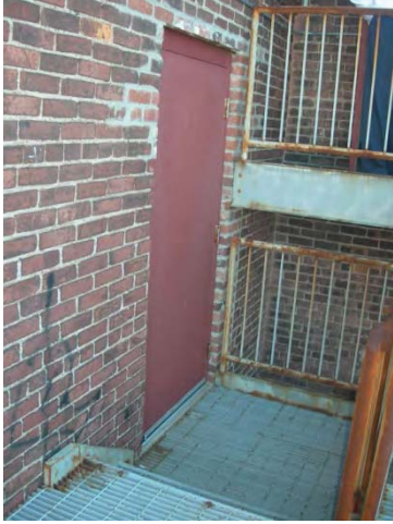
Photo 55- 2 nd floor – 2 nd means of egress
