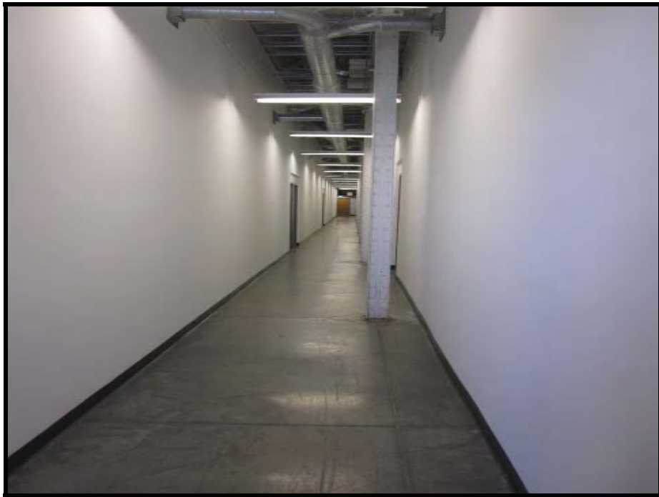
VIEW OF 2 ND FLOOR HALLWAY AREA
