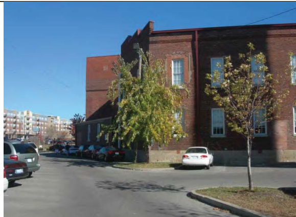
Photo 6 -.South SW elevation
