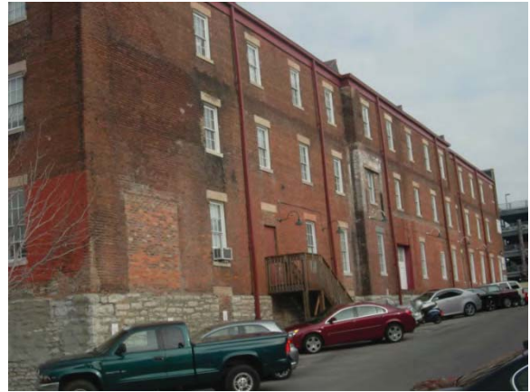
Photo 20 East SE elevation
