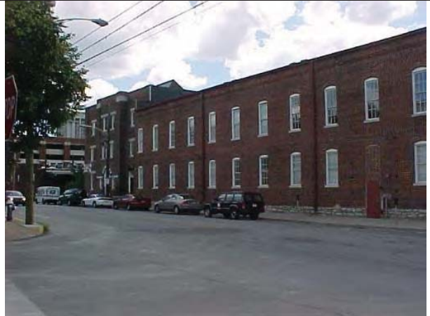
Photo 2 – North Elevation along Bolivar Street is generally in good condition
