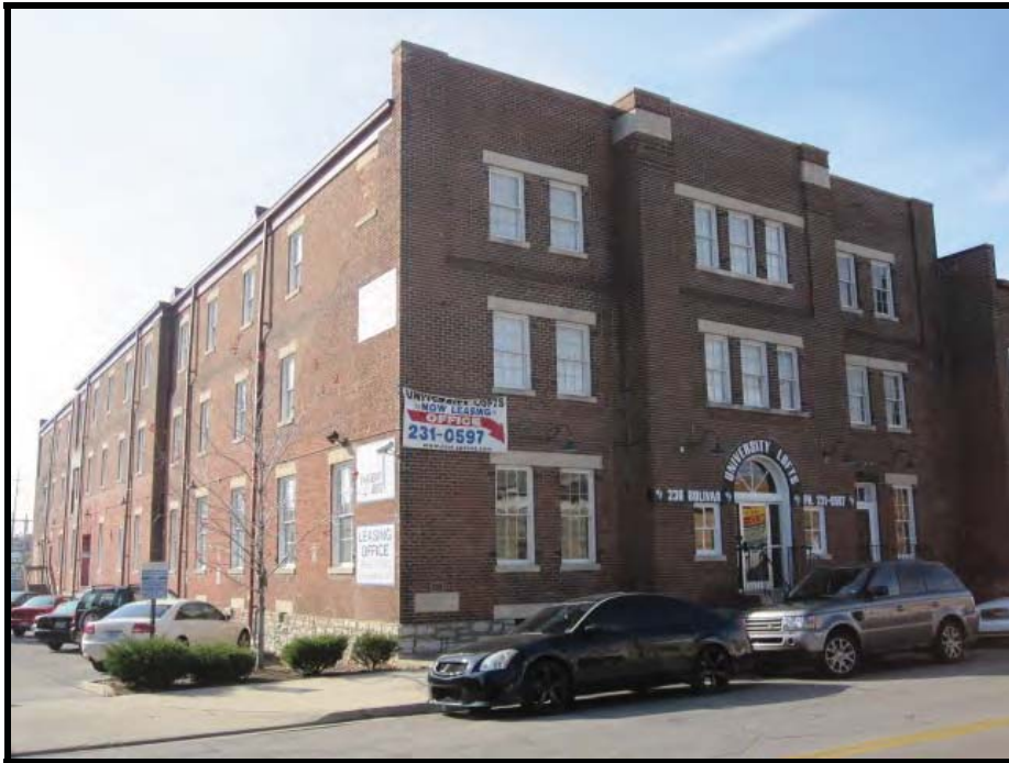
VIEW OF FRONT AND SOUTHEAST SIDE OF SUBJECT PROPERTY
