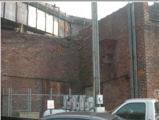
Photo 11- Electrical vault on left and boiler on right.
