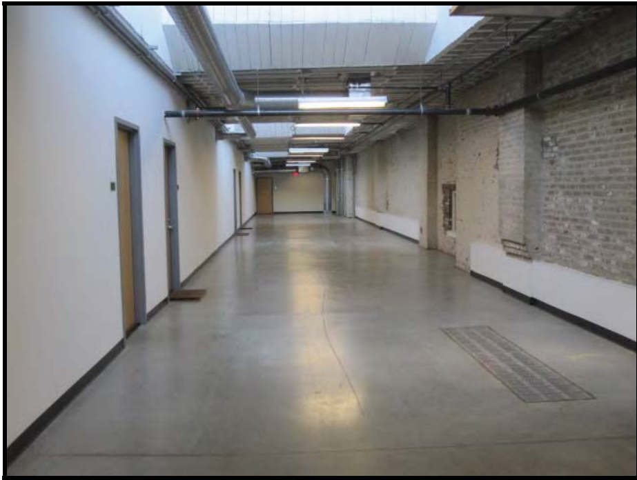
VIEW OF 3 RD FLOOR HALLWAY
