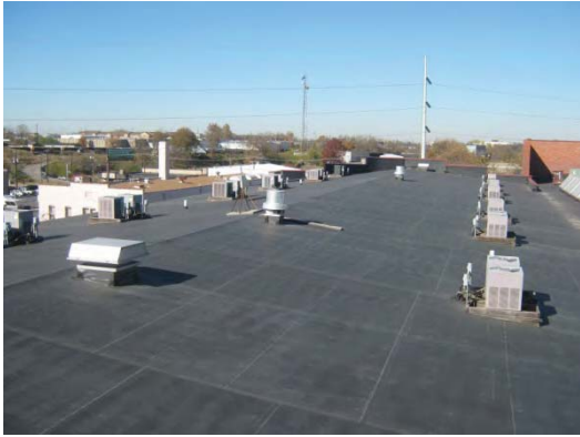
Photo 31- south side of roof
